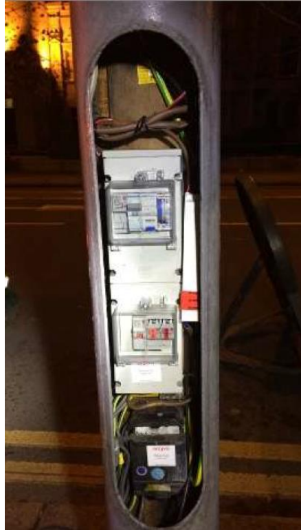
Internal Electrical Distribution
